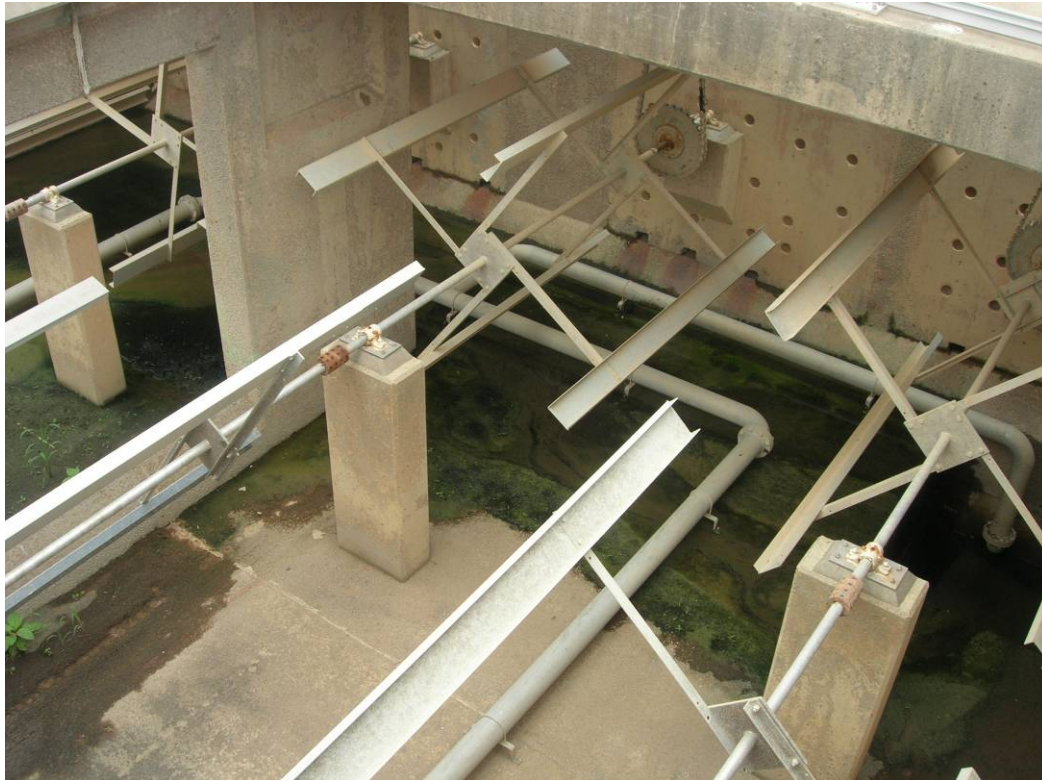
Chemical mixing paddles in front portion of sedimentation tanks at Alexandria AWWTP
