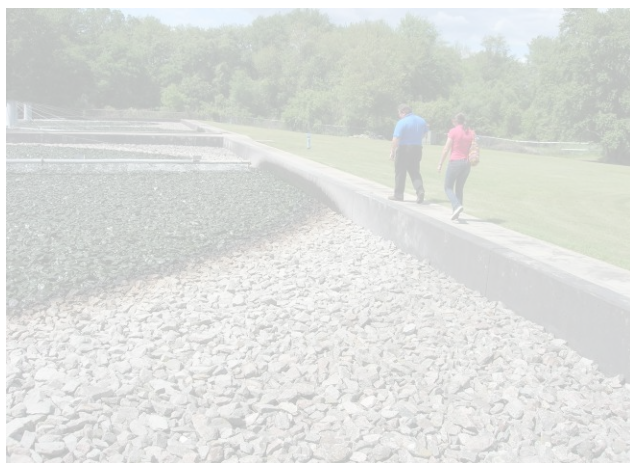
Trickling filters at Milford WWTP
