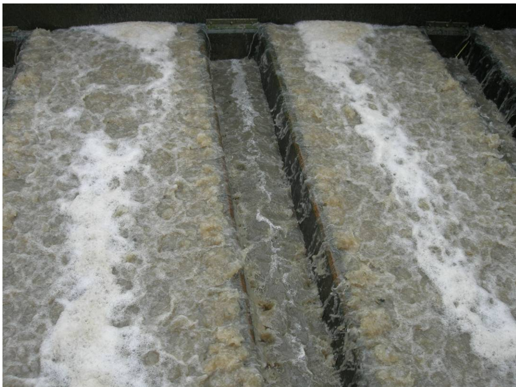
Bed filter undergoing backwash at Alexandria AWWTP
